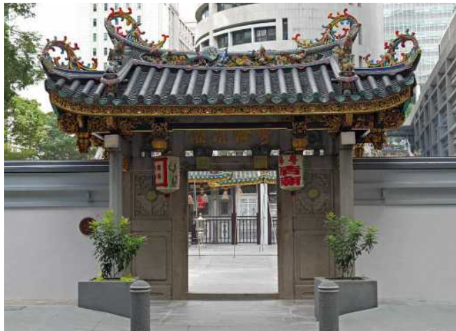
Restored entrance gate and reinstated boundary wall
