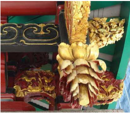
Intricate brackets and granite columns
