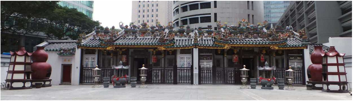
Front view of twin temple recovered and revitalised, complete with railings of original design and material
