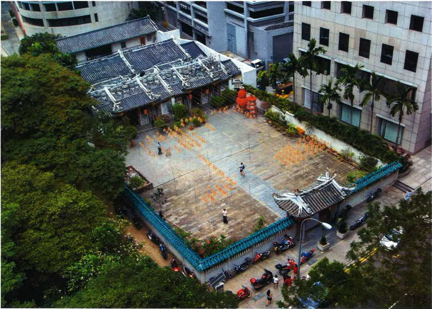
Boundary Wall – 2012. Balustrades were removed in the 1996 renovation.
