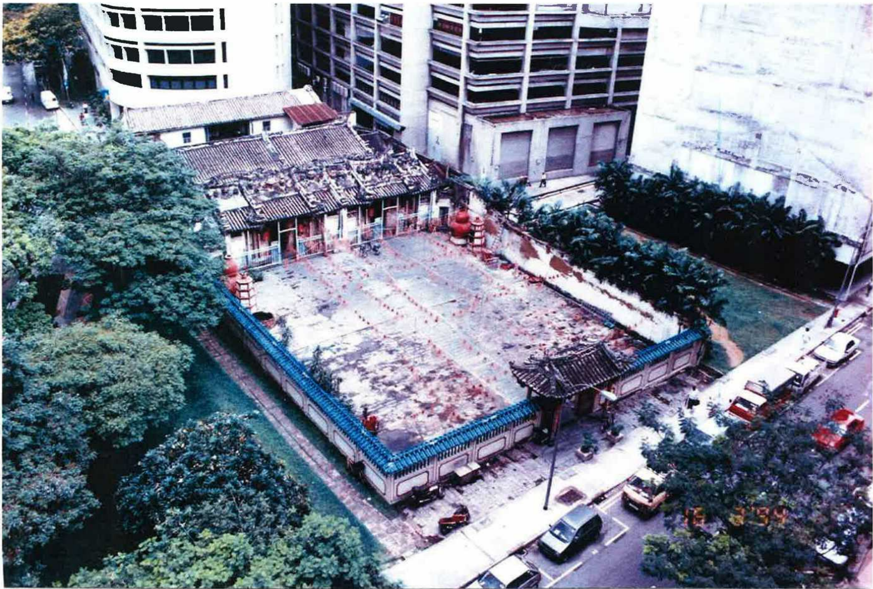
Boundary Wall – 1994. Balustrades at the twin temple.
