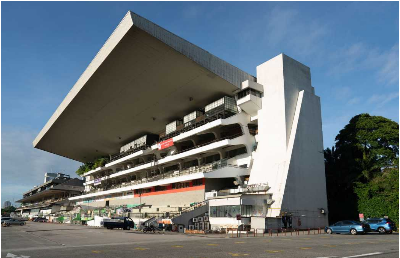
Figure 4.2 North Grandstand in 2021
