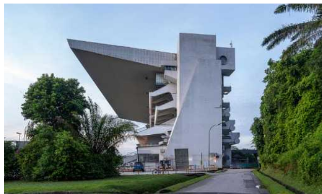
Figure 8.4: Existing view looking south to the North Grandstand.
