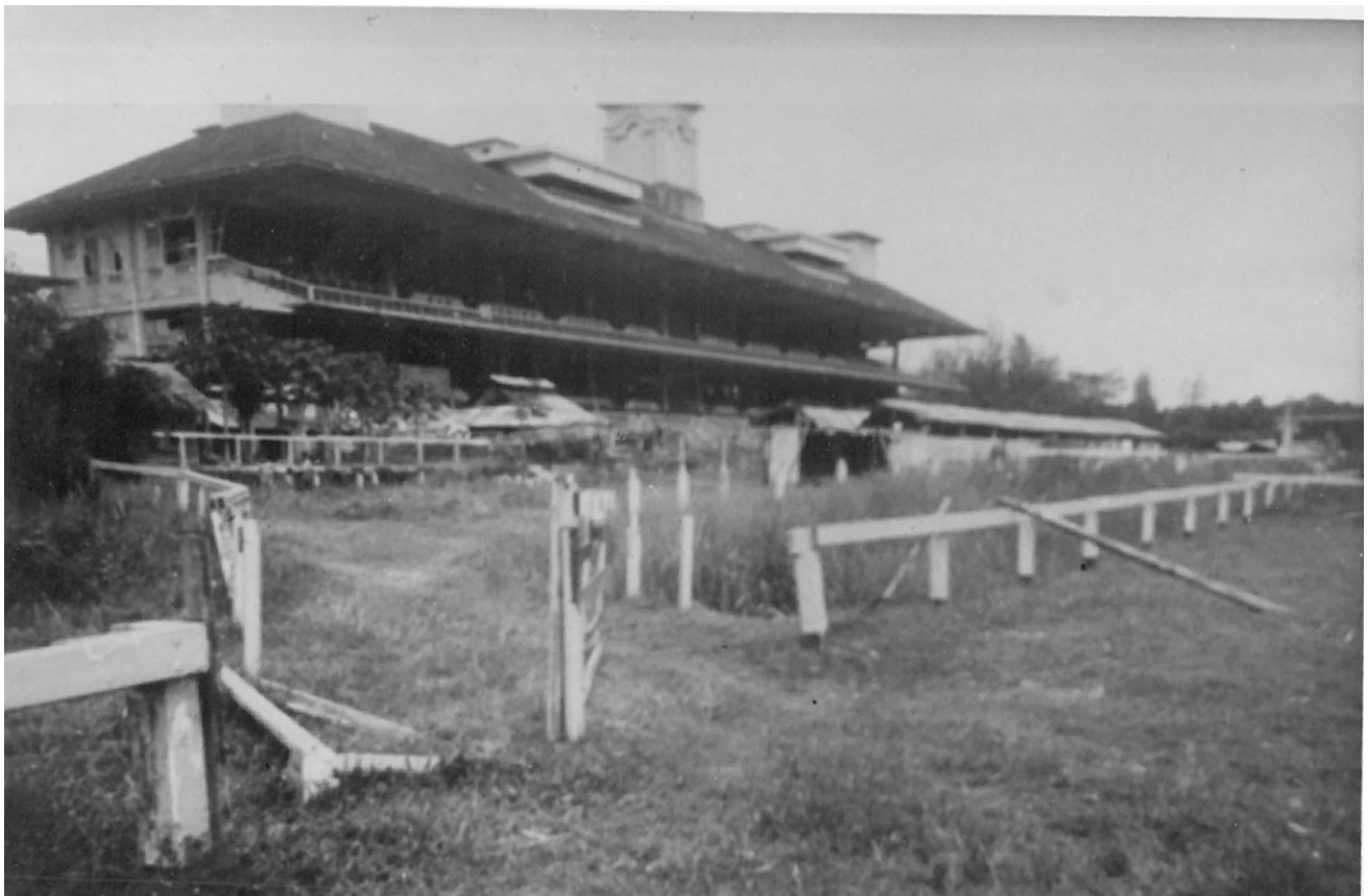
Figure 4.21 Post War view of South Grandstand. (Source: Mark Bailey)
