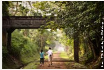
The Rail Corridor has been transformed into an inclusive community space that retains the unique identity of the former railway line.
