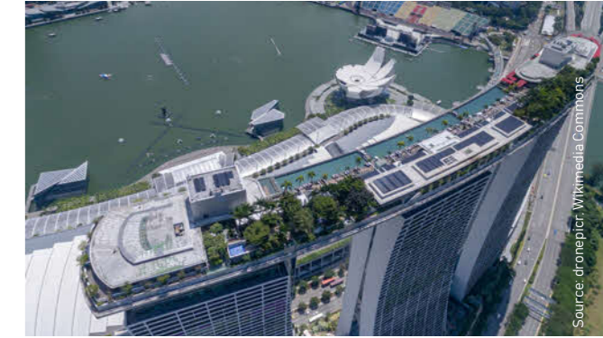
Rooftop public space at Marina Bay Sands made possible with district cooling systems which remove the need for individual cooling towers
