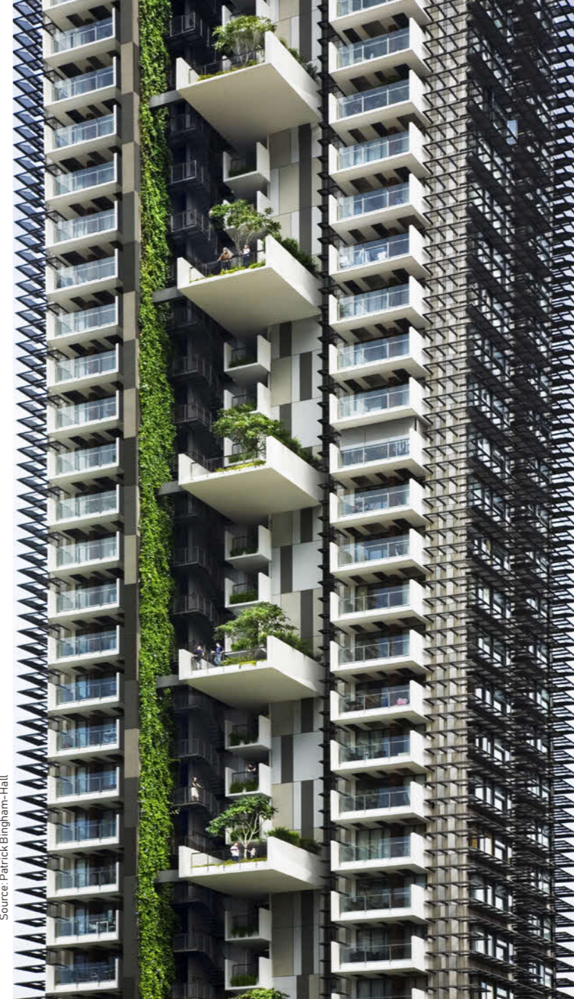
Shaping of building form to promote wind flow at street level
