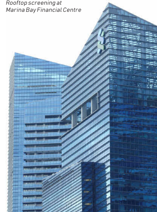
Integration of services into the building envelope at CapitaGreen
