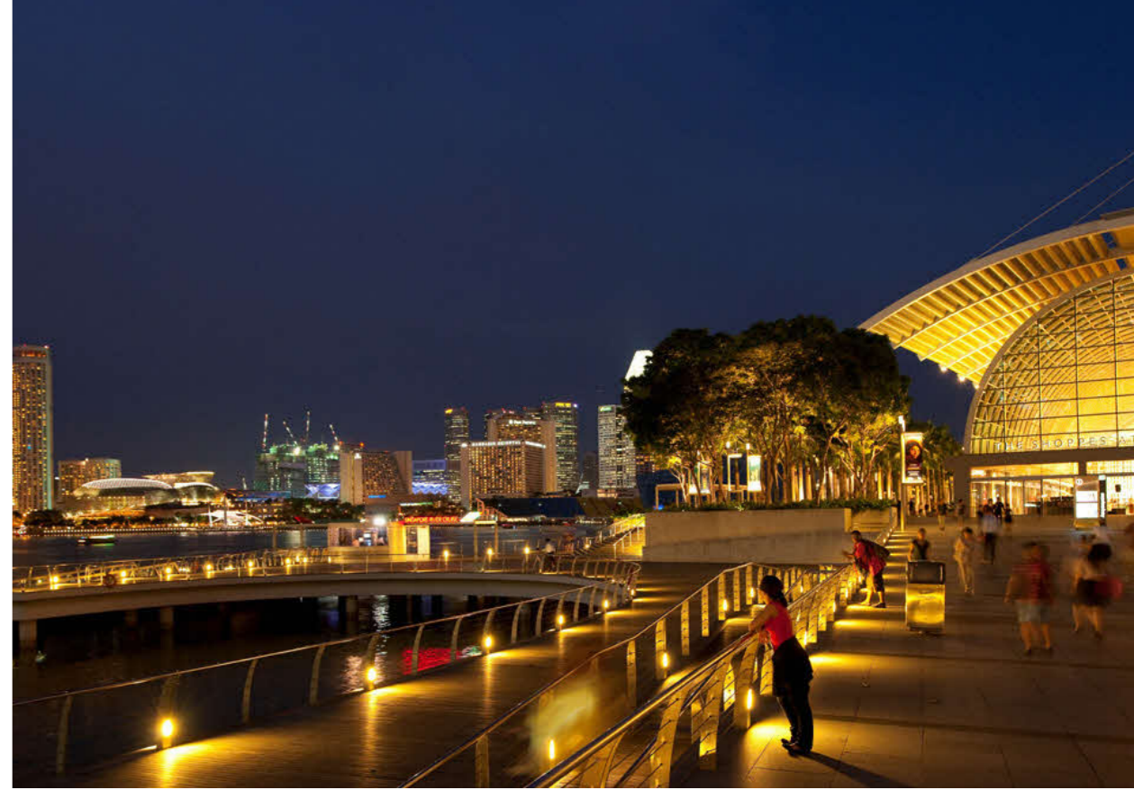
Sensitive indirect lighting to minimise glare in the public realm, Marina Bay
