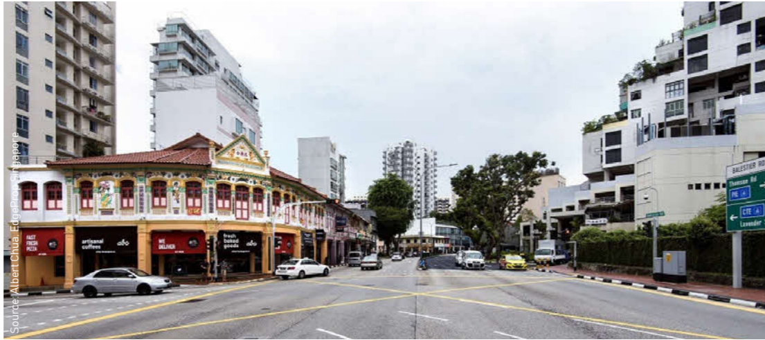
Mix of old and new along Balestier Road
